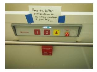
The difference between a "Lift" and an "Elevator" is primarily in the way they operate from the inside. A lift requires that you hold down the button until you have reached the floor of your destination. An elevator just has the need for one press of the button. The lift at Torg brewery was already part of the building when they purchased and offered a great way for people with wheelchairs, or those unable to climb the stairs to get to the second floor. But it's a **Lift**, not an elevator.
